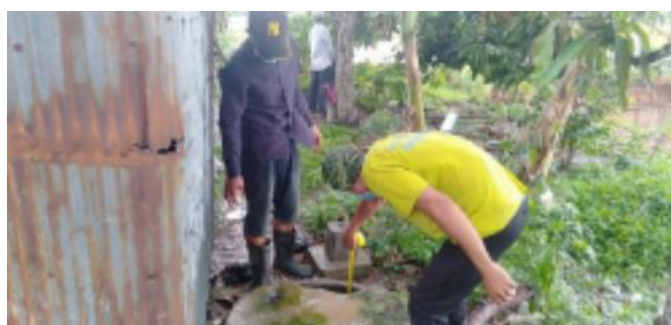
Figure 2: Measuring the sludge level within a pit
